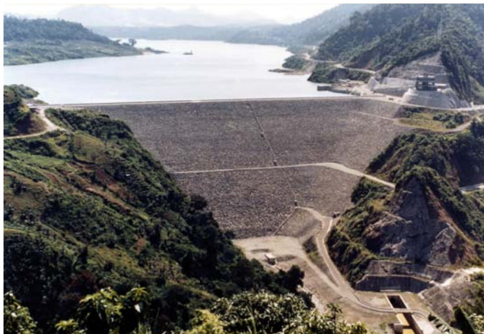
Concrete Faced Rockfill Dam (126 m high)
