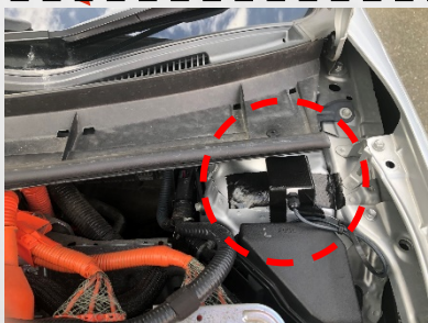
Installation location of upper sensor
