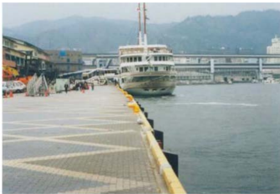
Example of damage to a mooring wharf after the 1995 Hanshin-Awaji Earthquake (The wharf appeared to be sound, but the steel sheet piles had buckled)
